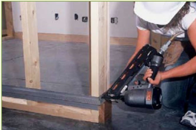
Figure 4-1: Using nails with a nail gun is the fastest way to fasten the UMB to wood.
