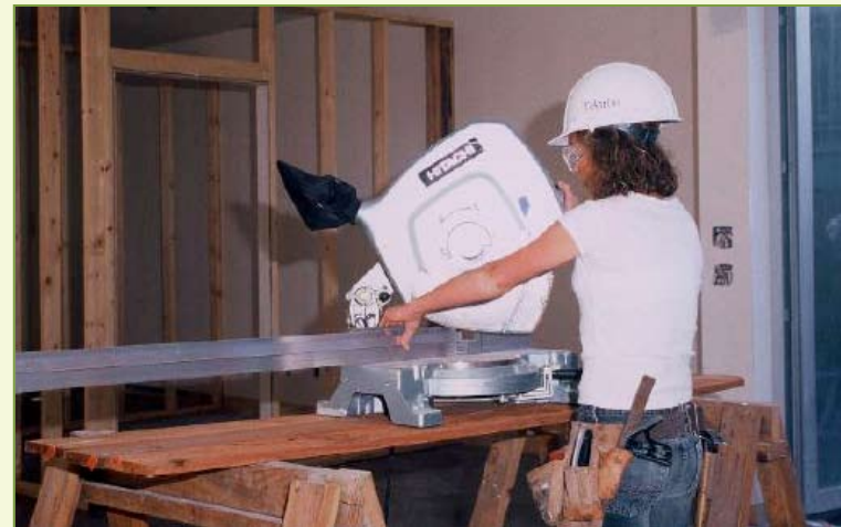
Figure 3-1: Feed the chop saw blade slowly and steadily through the aluminum UMB.
