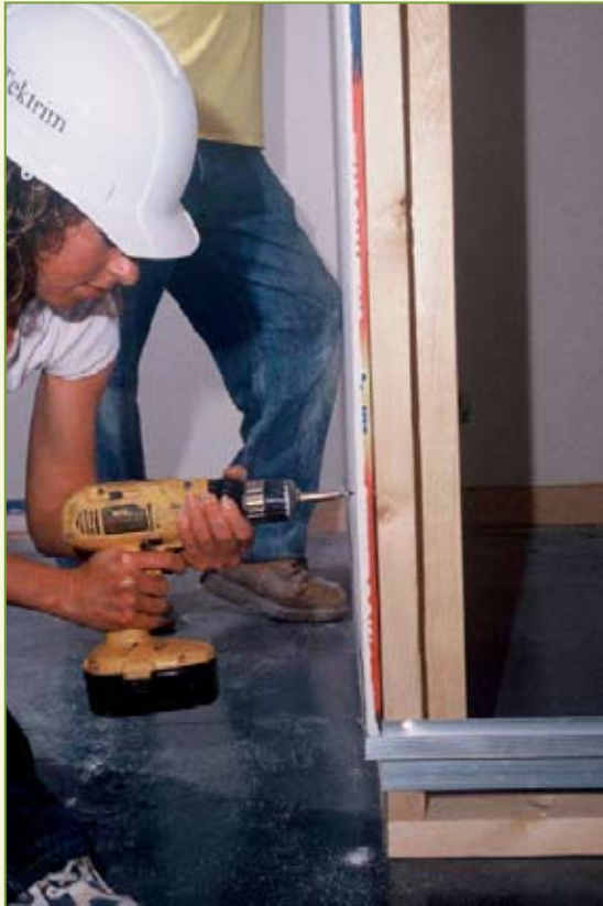
Figure 5-6: Fasten the drywall to the framing conventionally.
